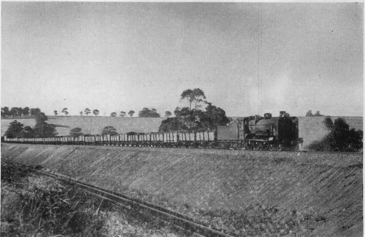
A Train Load of Briquettes on a Newly Duplicated Section of the Gippsland Line.
